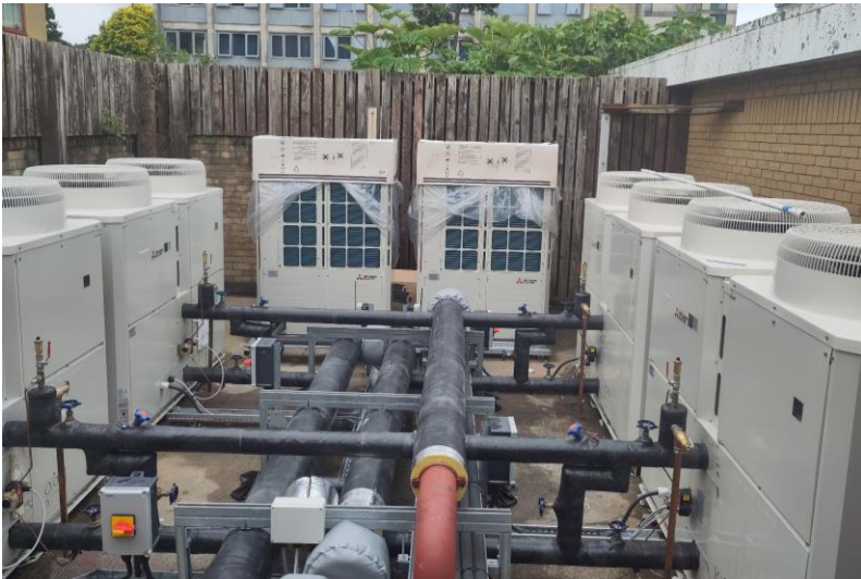
Haldane Building, air source heat pump
